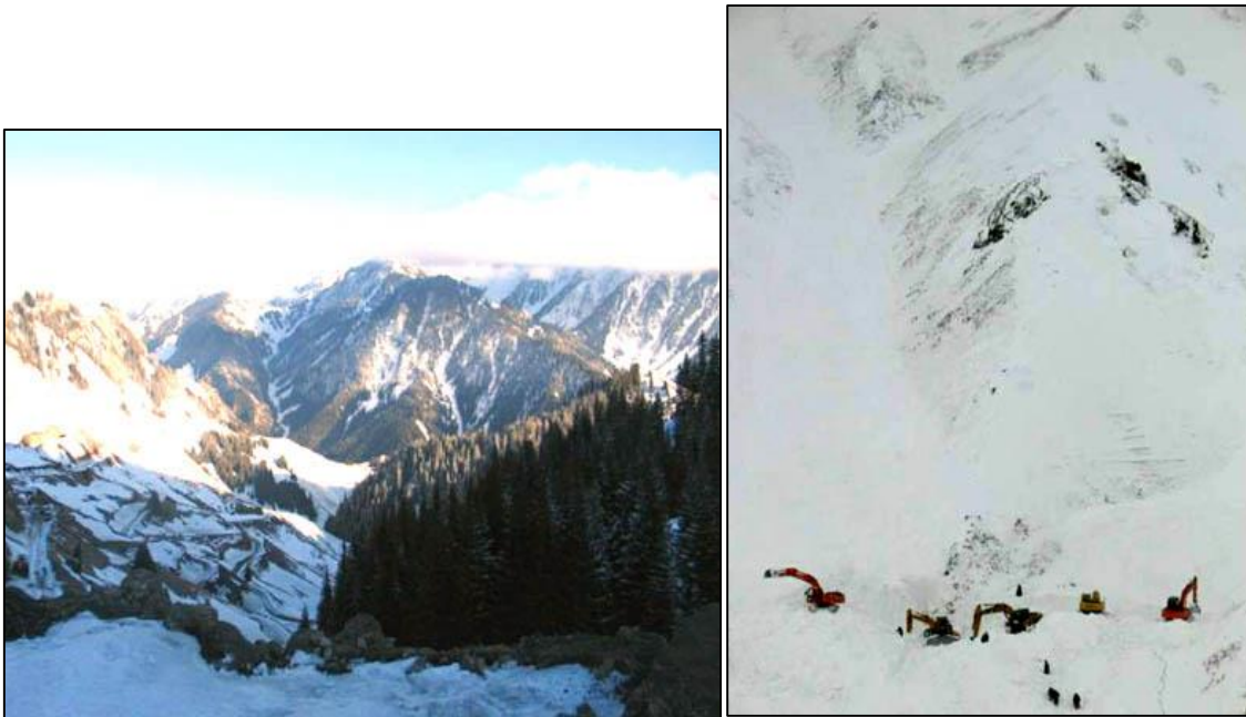
Fig.1.1 The mountainous section where a tunnel are under construction (left) and grabs clear the snow (right) (from www.chinaview.cn ).
