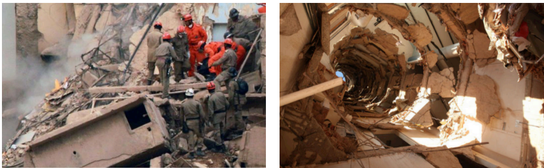
Figure 4.12 Bypasses in Layout Adaptation Resulting in Building Collapse: Rio de Janeiro, left (Freitas and Nunes, 2012), and Sao Paulo, right (Queiroz, 2012)
