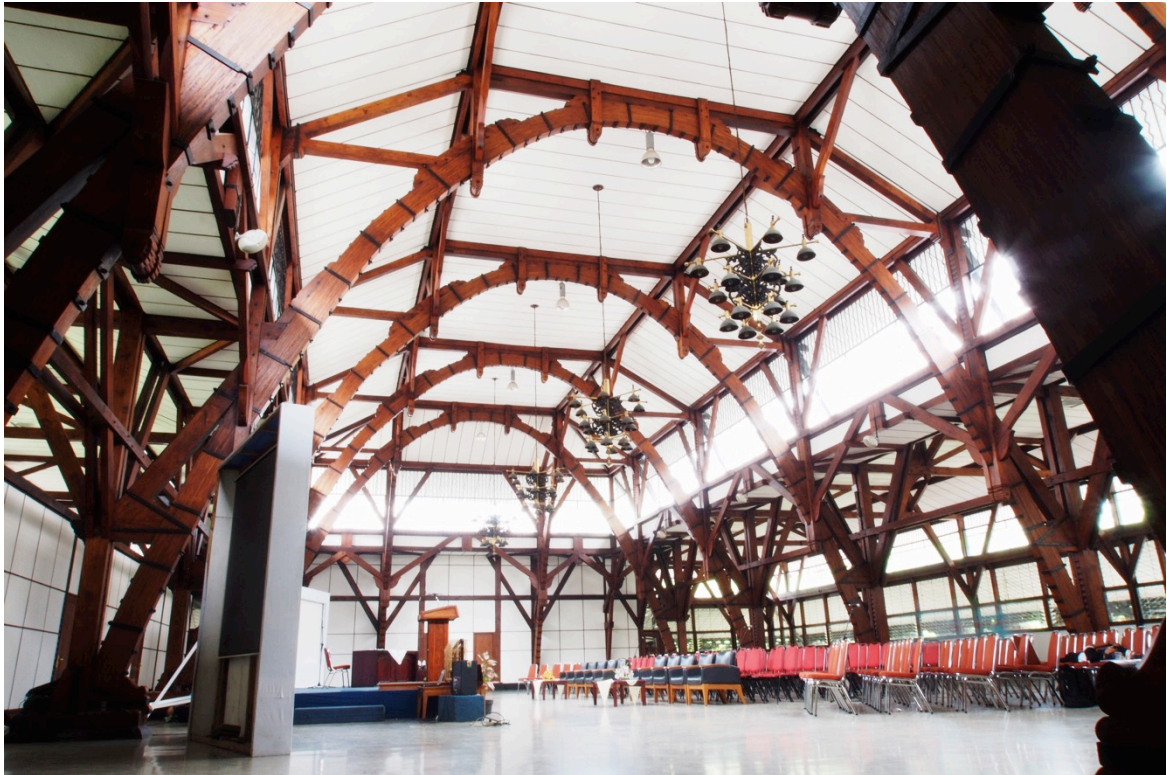
Figure 3.2. One of the 1920's university buildings in Indonesian in which uses laminated-teak for its main construction.
