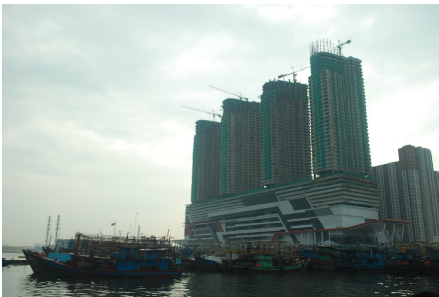
Figure 2.4. Photo of tower buildings under construction along the Jakarta coast Source: Author
