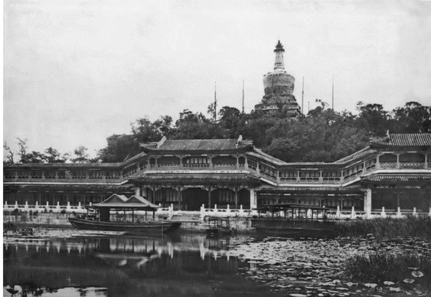
Figure 4-19 Garden Space of Bizhao Building[碧照楼]
