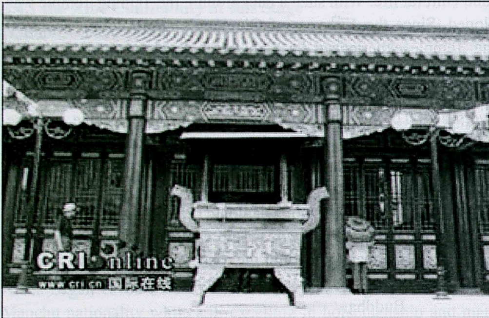
The Main Hall of Taiping Temple
