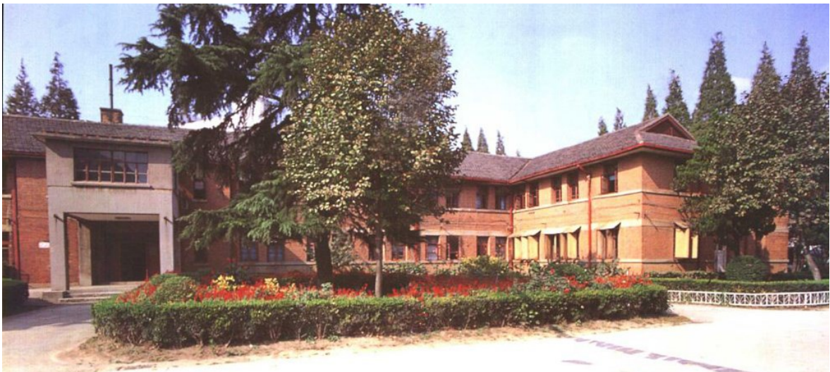
Figure-3-11 The Office Building of NO.18
