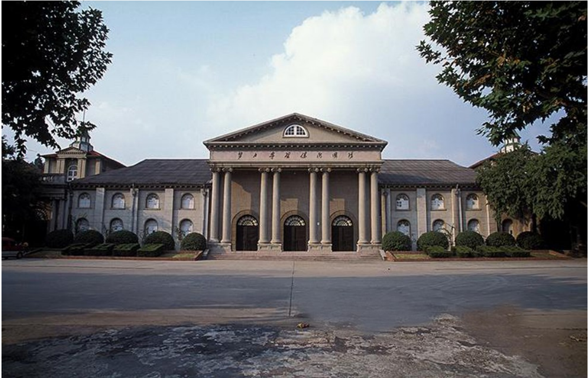
Figure-3-10 The Office Building of NO.8
