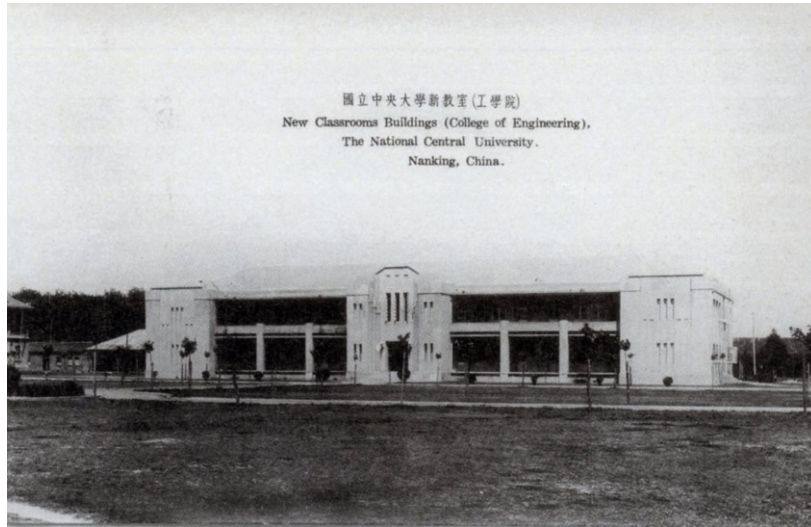
Figure-4-8 The Main Square and the New Classroom Building (No.7)
