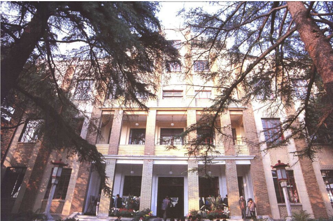
Figure-3-5 The Office Building of NO.1
