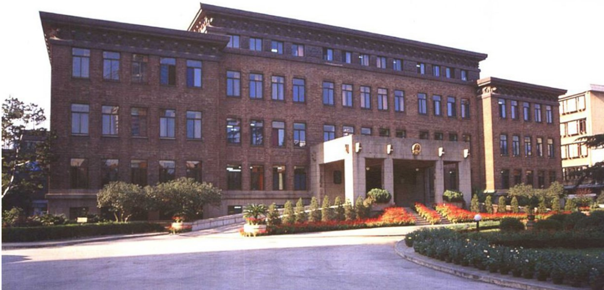
Figure-3-9 The Office Building of NO.7
