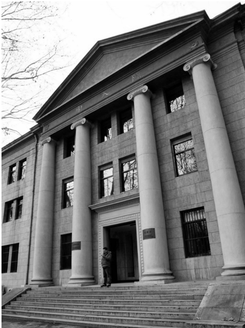
Figure-4-9 The Main Entrance of the Biology Building (No.3)
