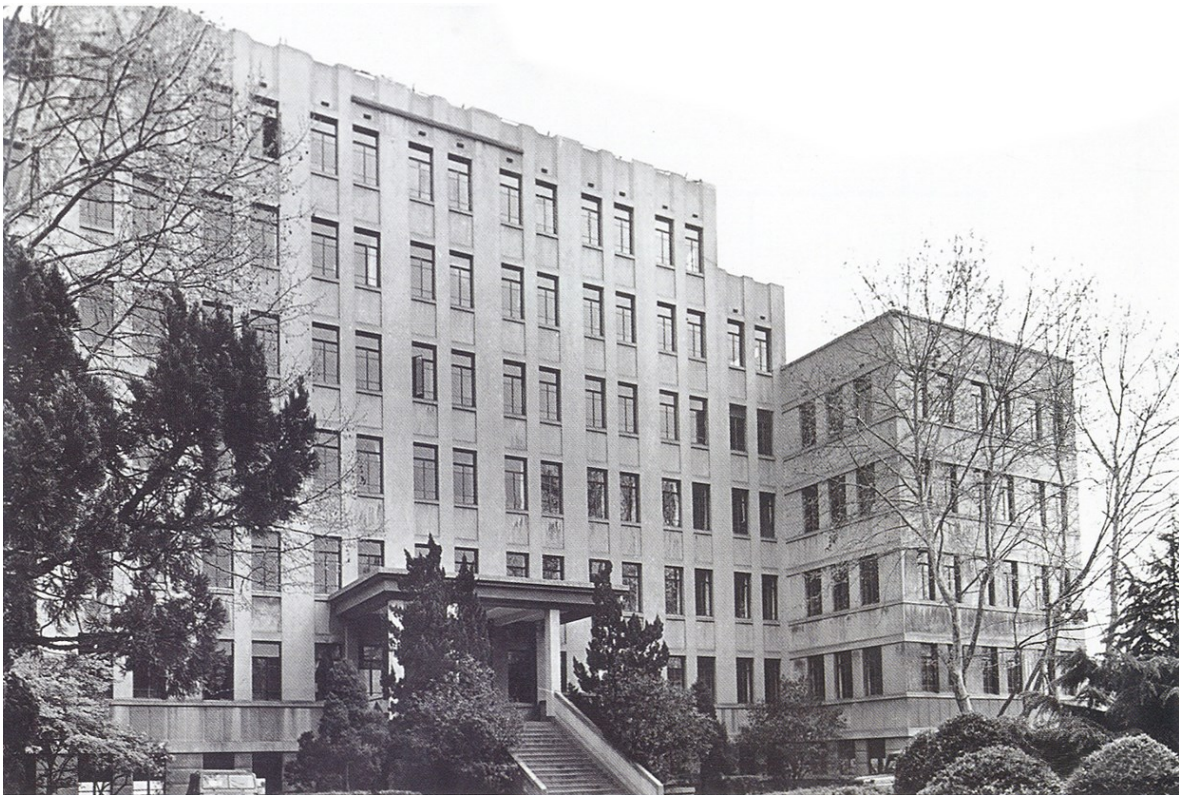
Figure-3-17 The Office Building of NO.24
