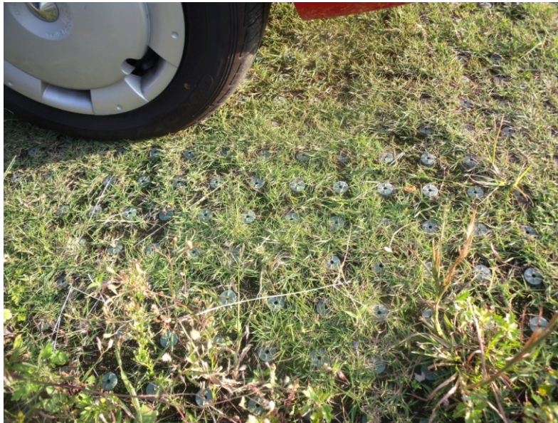
Appendix 12: Storm water management: reinforced lawn parking to allow rain water to infiltrate where it falls in Koshigaya Laketown (source; author, field survey Koshigaya Laketown).
