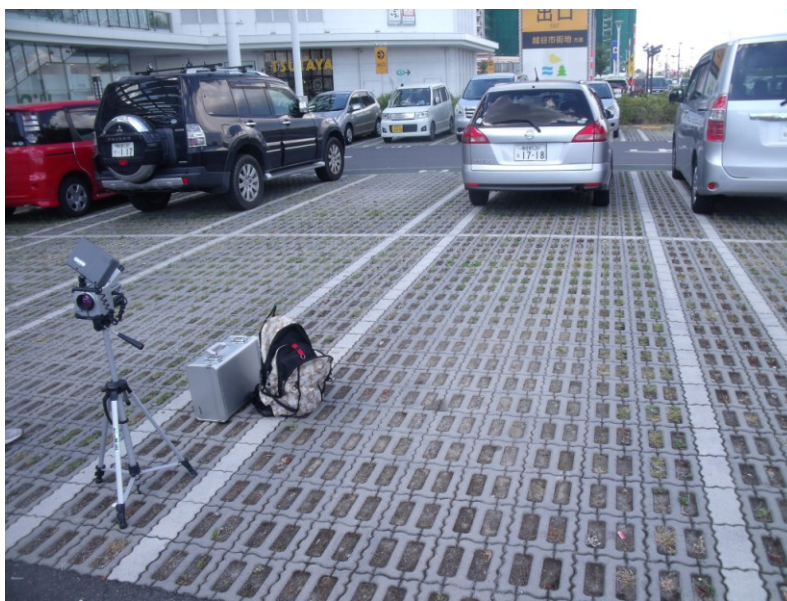
Appendix 13: Storm water management: hollow concrete block parking to allow rain water to infiltrate where it falls in Koshigaya Laketown (source; author, field survey Koshigaya Laketown).
