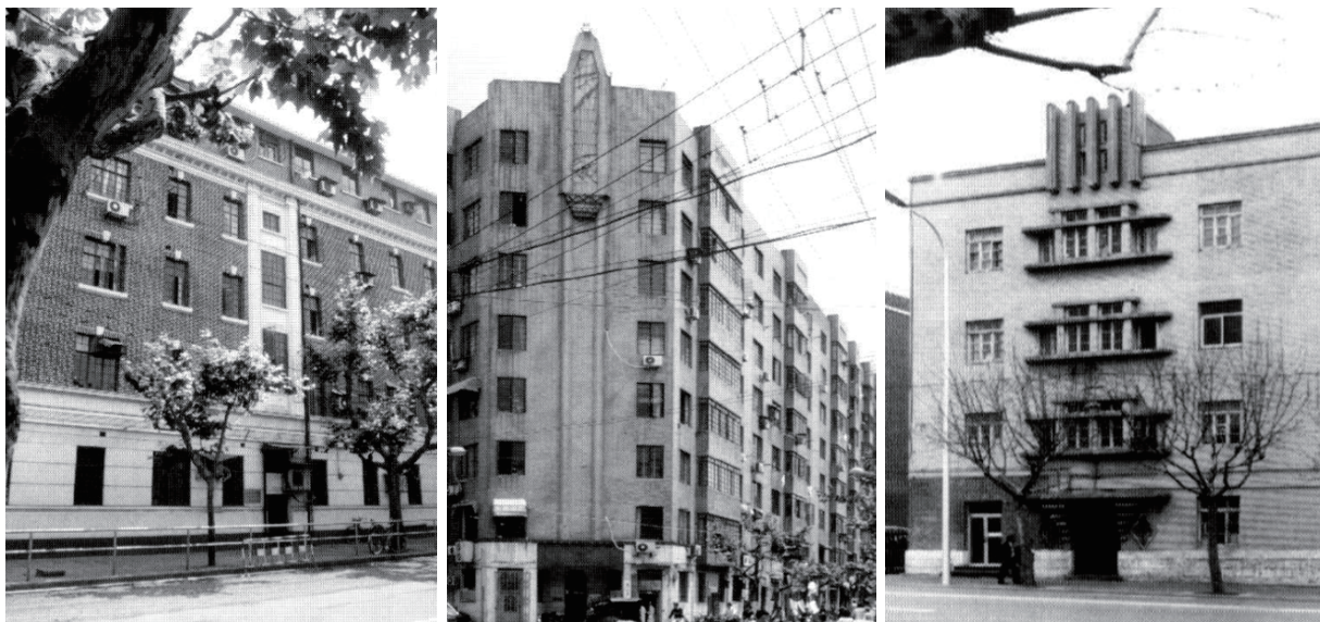
Figure 3.12 Individual multi-story apartment buildings in different cities (from Lu Junhun 2001, 92)
