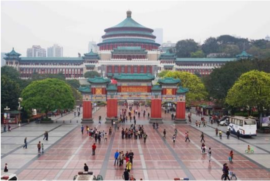
Fig.6-3-7 Chongqing People's Auditorium
