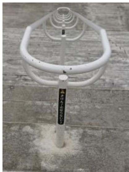
Fig.4-4-7 Warning on Handrail
