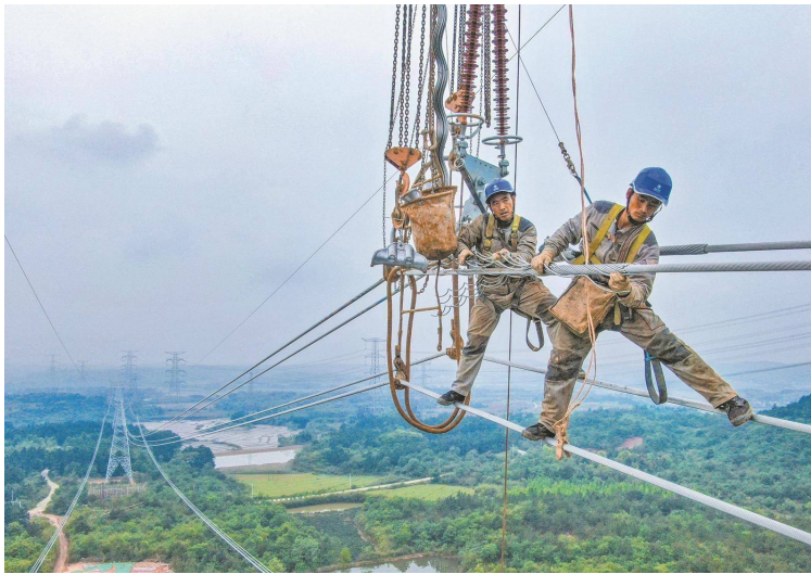
Figure 2-6: Manual inspection along transmission lines.
